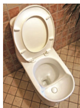
Fig. 7.12 – Urine diverting flush toilet. Image source: www.Dubbletten.nu
