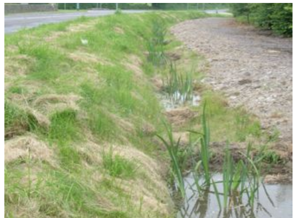
Fig. 9.6 – Roadside swale in north Cork, with earthen check-dams and pocket pools planted by volunteers as part of local community scheme.
