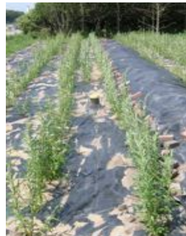
Fig. 7.9 – Newly planted zero discharge willow system in Denmark, showing three rows of cuttings on either side of the central covered spreading pipe. Outer bund work due for completion the following February.
