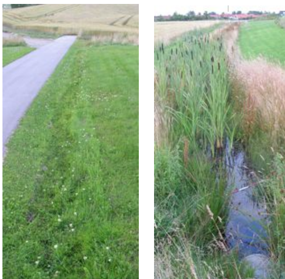
Fig. 9.7 A & B – Two swale examples from a stormwater drainage system in Denmark for village urban runoff. Dry grassed swale (L) and wetland planted swale (R) both filter water en route to a stormwater wetland lower in the catchment.
