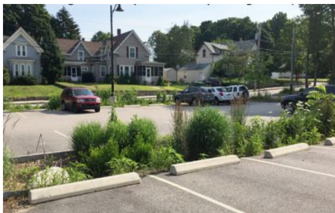
Fig. 9.9 – Sunken rain-garden strips between parking rows (below). Image source: www.ecolandscaping.org
