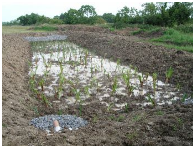
Fig. 7.3 – Newly planted wetland system for single dwelling, filled with clean water for planting and plant establishment.
