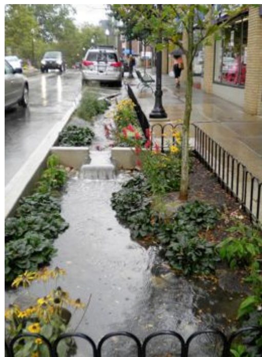
Fig. 9.8 – Rain-garden during downpour (R) Reproduced with permission from State College PA, USA. www.statecollegepa.us/345/On-Street-Rain-Gardens
