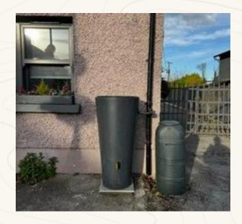
Harvest rainwater from a roof by connecting a diverter to a down pipe to divert water to a garden pond or planter. Visit https://www.wikihow.com/build-arainwater-collection-system for DIY tips.
