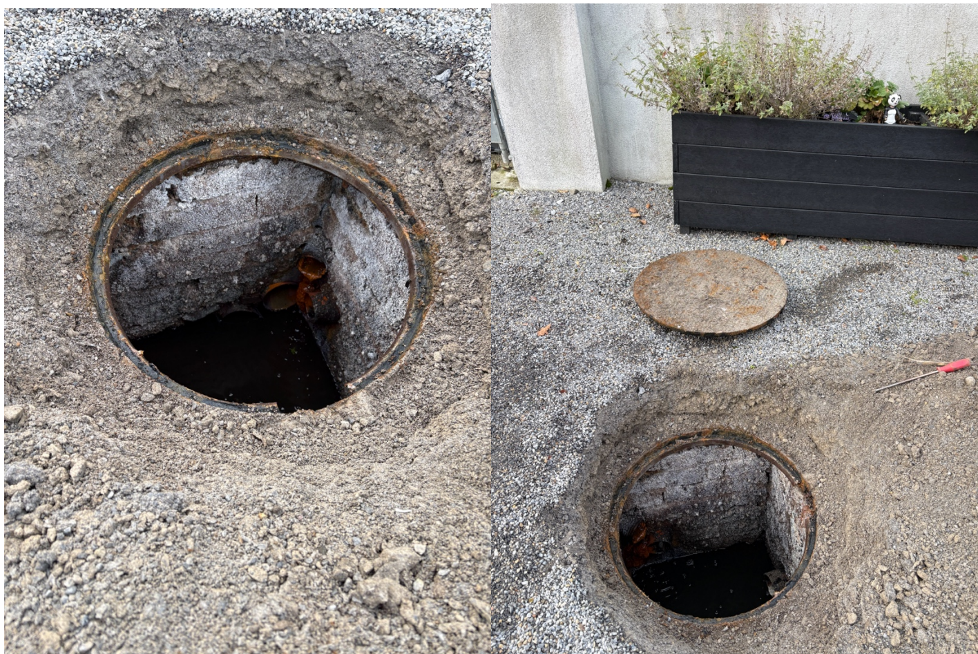
The manhole in the public area.
